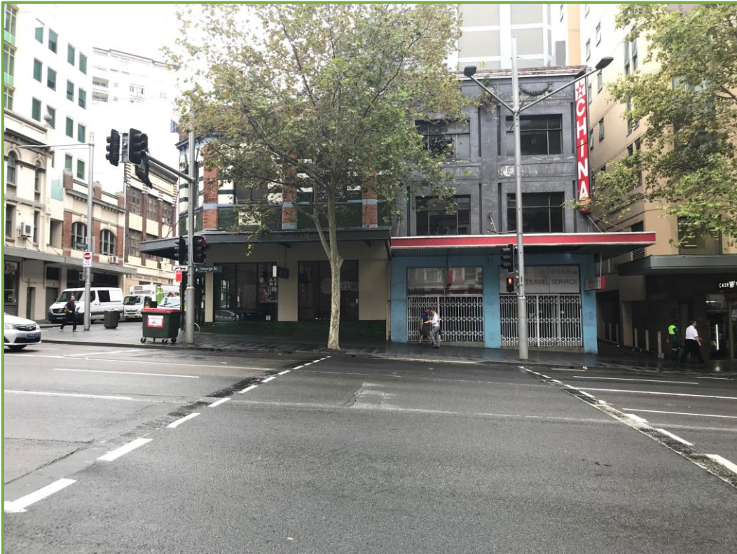
View looking west across George Street at the site.
